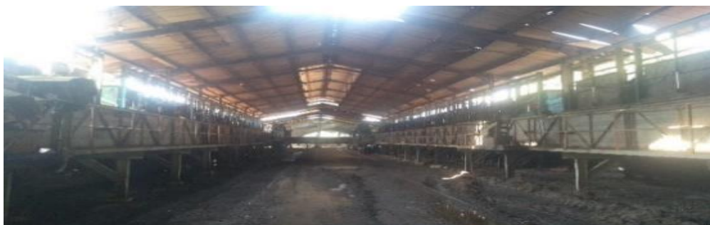
Figure 3. Station Loading Ramp
